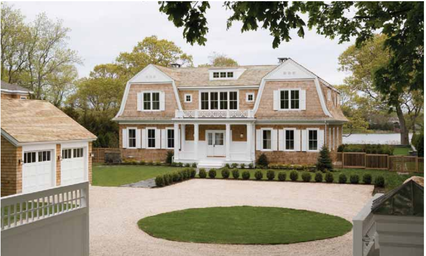
82 Ferry Road on Sag Harbor – Completed and sold by PCH in Spring 2008.
